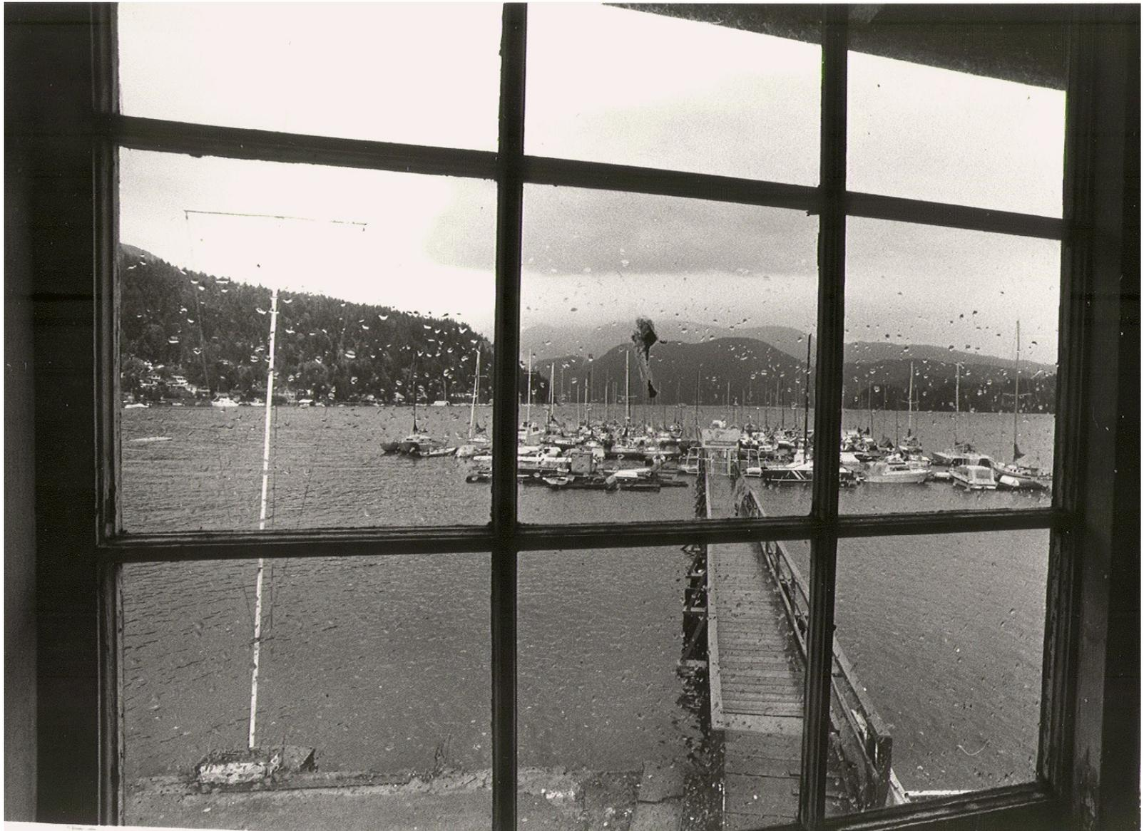
The view of the docks. Note no hand rail along the water's edge, the old pier with wooden hand rail, and the gate located at the top of the ramp. The gate was relocated to the shoreward end of the pier before being replaced with the aluminum one in 1998.
