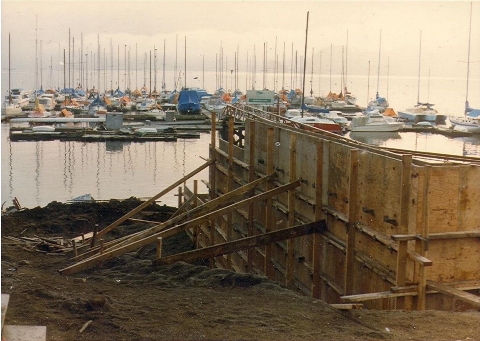
*With erection of the concrete forms progressing quickly.*
