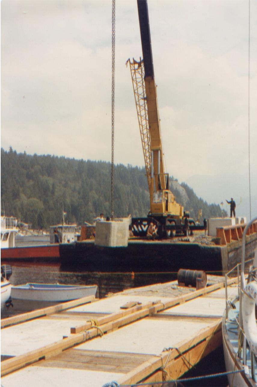
Placing the anchors for A Dock. The new dock required twelve by 12T concrete blocks. Summer 1980.
