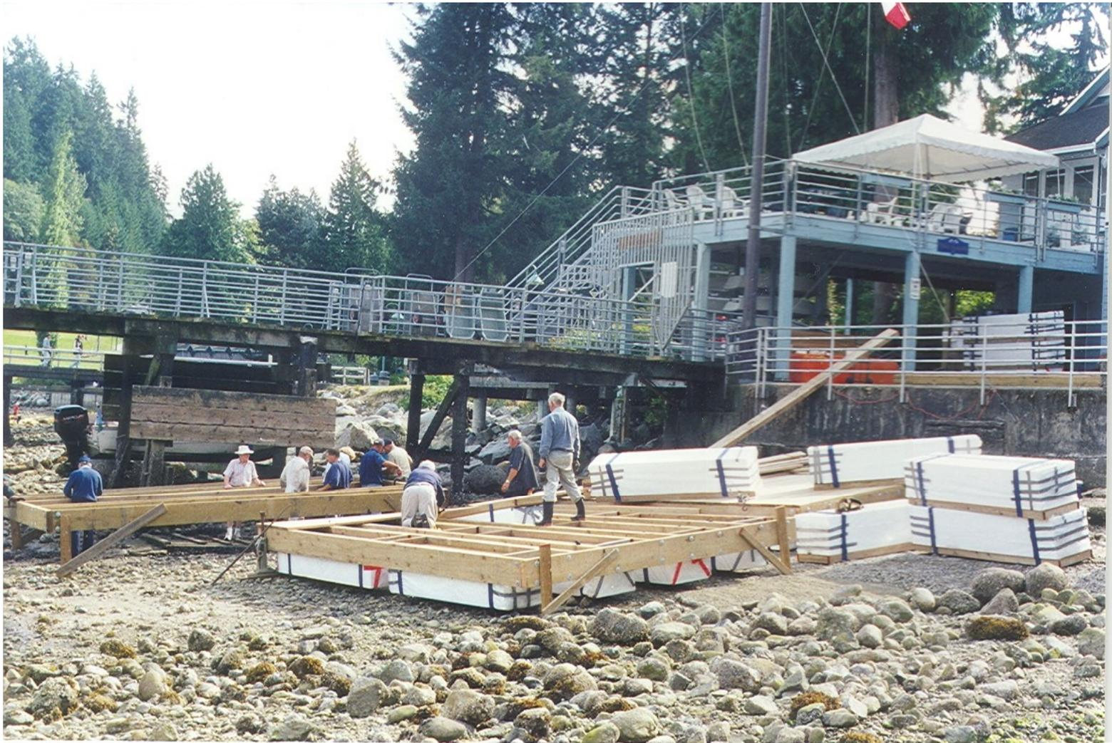
The three modules that make up the ramp dock under construction. A similar design was adopted for all docks constructed by the club. All lumber is 3" x 12" full dimensioned treated fir, with a 2" x 6" treated fir deck. The floatation consists of 30" x 60" X 20" deep plastic-wrapped polystyrene.
