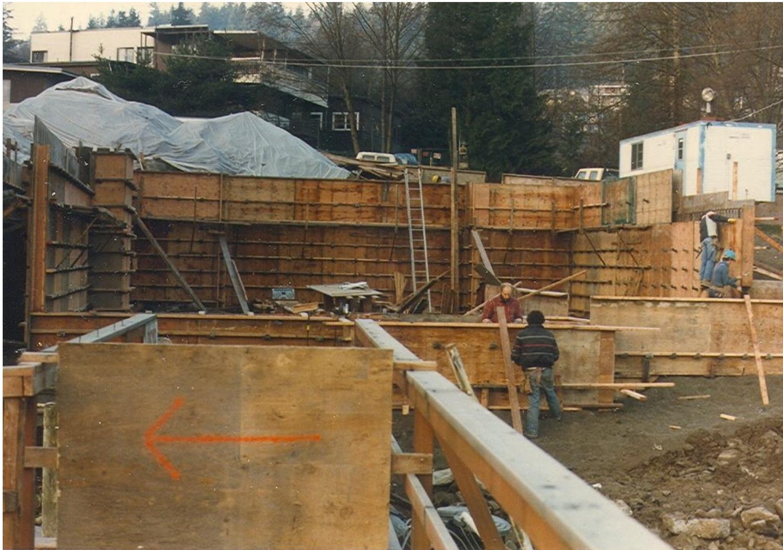
*The forms for the basement concrete foundations -
