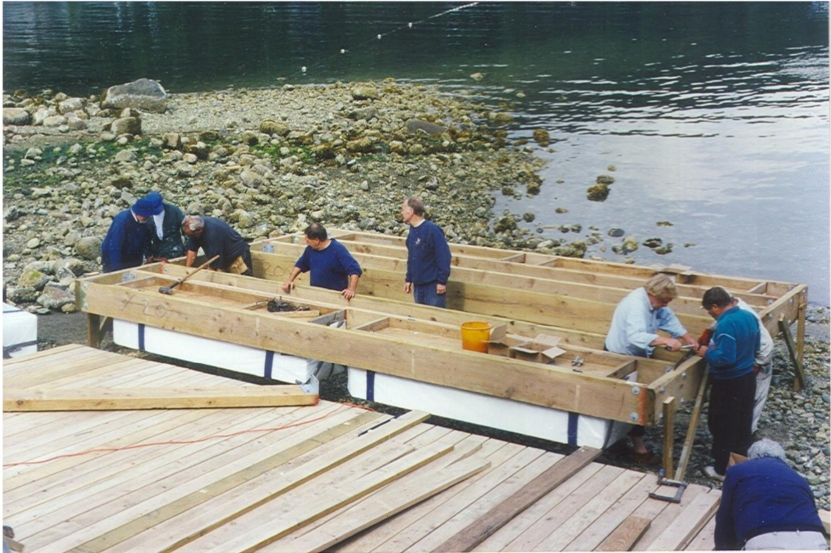
*The first module is almost complete. Work is underway on the second module as the tide falls.*
