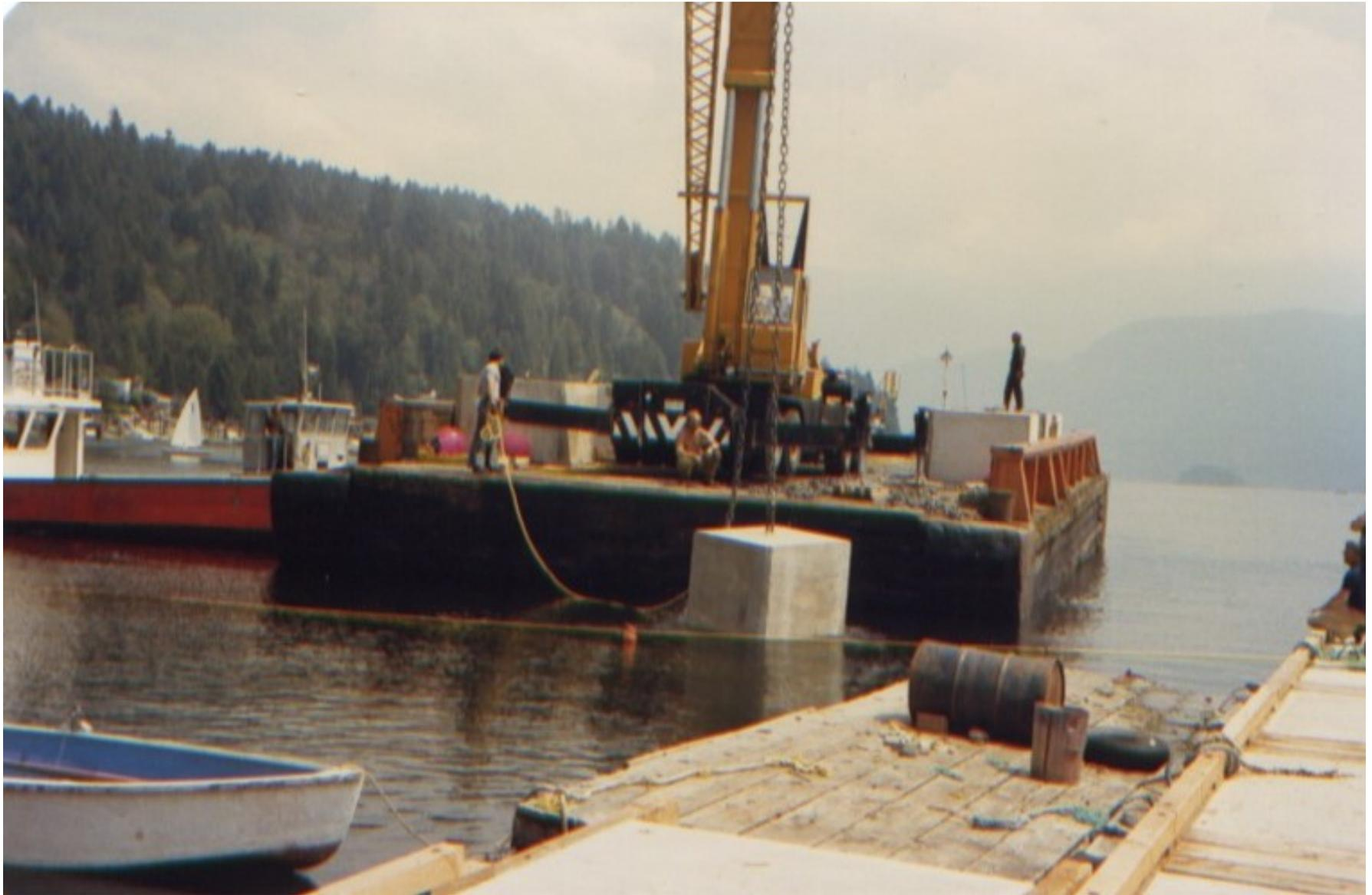
*A 12T block being carefully lowered on 7/8" long link chain.*
